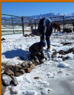
Jerry Allen, SCD IWM, shows students how to stabilize ditch banks to reduce soil erosion.
